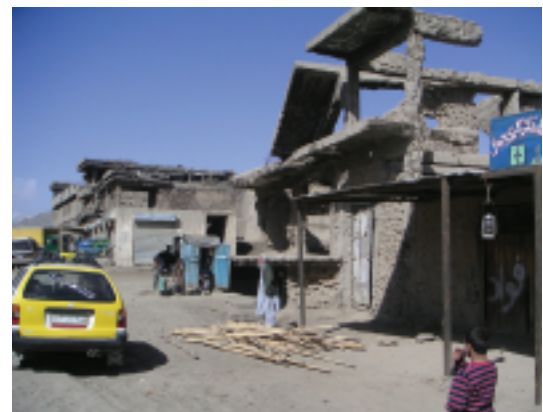
Destroyed house in Kabul
