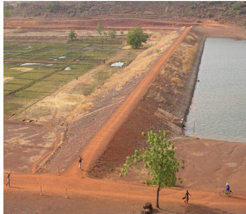
Dam constructed for small-scale irrigation
