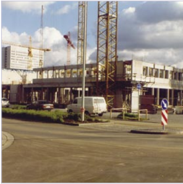
Setting up a Center... ZEF building in 1989
