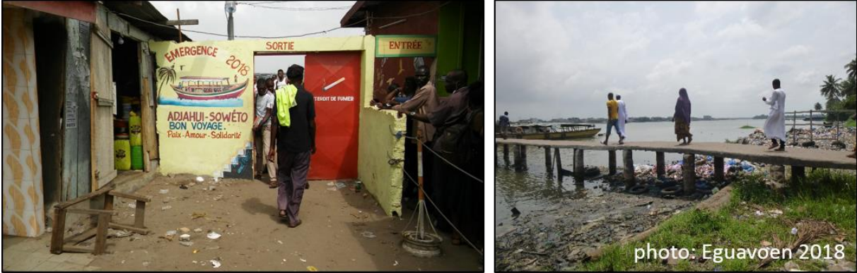
Figure 7: Quay Hôpital Nord
