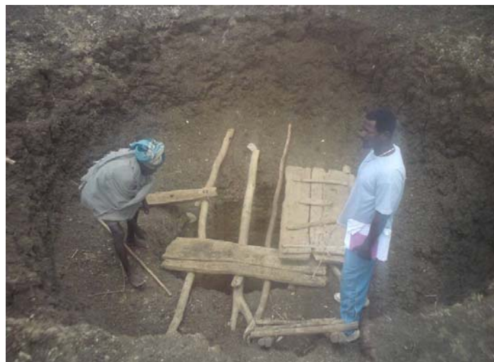
Figure 5: Construction of a V-shaped well
