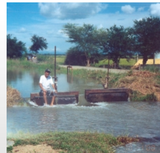
Irrigation facilities in the Philippines.
