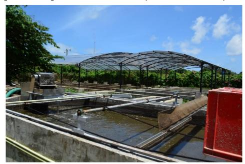
Figure 6: Treating wastewater in a small-scale plant in Colombo Municipal Area
